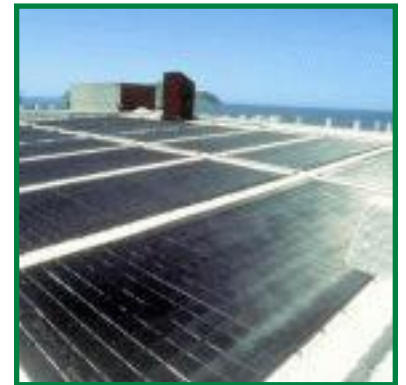
Solar panels on a roof
